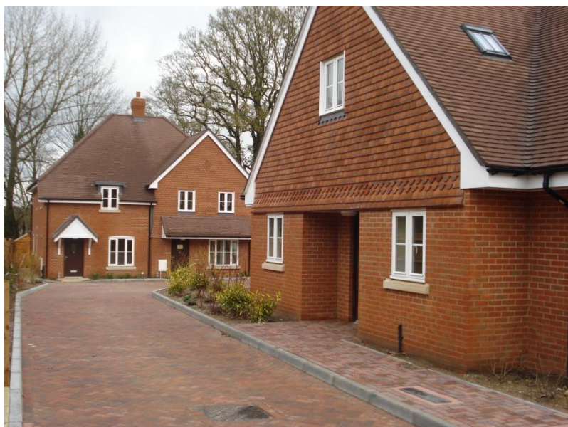
Photo 5: 11 new affordable homes at Arnold Close, Dunsfold for people with a local connection (part rural exception and part s.106 site), completed in 2010, owned and managed by English Rural Housing Association.
